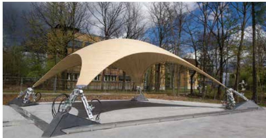
Figure 10. Stuttgart SmartShell with one of the three active supports (support 1 from figure 8) in foreground (photo Bosch Rexroth).
