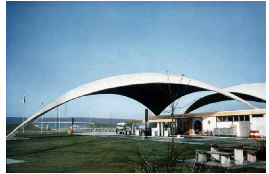
_ Figure 3. Heinz Isler, Service station Deitingen-Süd, a thin concrete shell with a geometry based on the inversion of a hanging cloth (ILEK archive).
